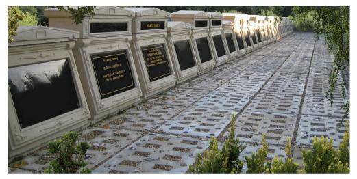
One of **welters**<sup>®</sup> most understated products is our grass mats. The grass mats are laid in similar style to paving stones but the holes within the structures can be seeded for grass or filled with gravel or another dry material.
