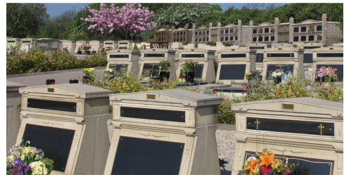
Their development of the mausolea interment unit allows **welters**<sup>®</sup> to provide both front and side charging options as shown. These units dominate the section and are also utilised as retaining structures, allowing the ground level to change. The ground level behind the mausolea is ~1m higher than that at the front.
