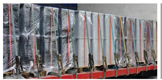
Once the off-site assembly of the parts is completed, they are securely packed and loaded on the appropriate vehicle for delivery to site.
