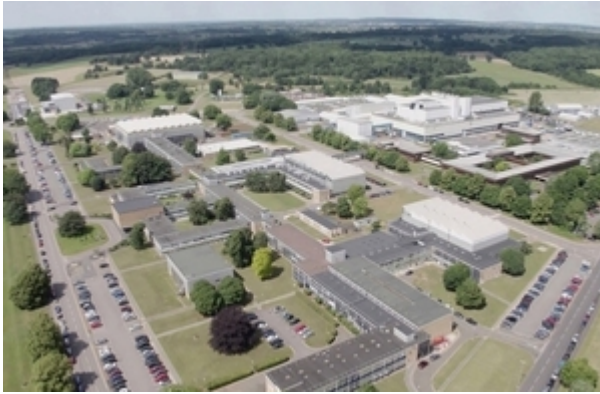
Culham Science Centre – headquarters of UKAEA
