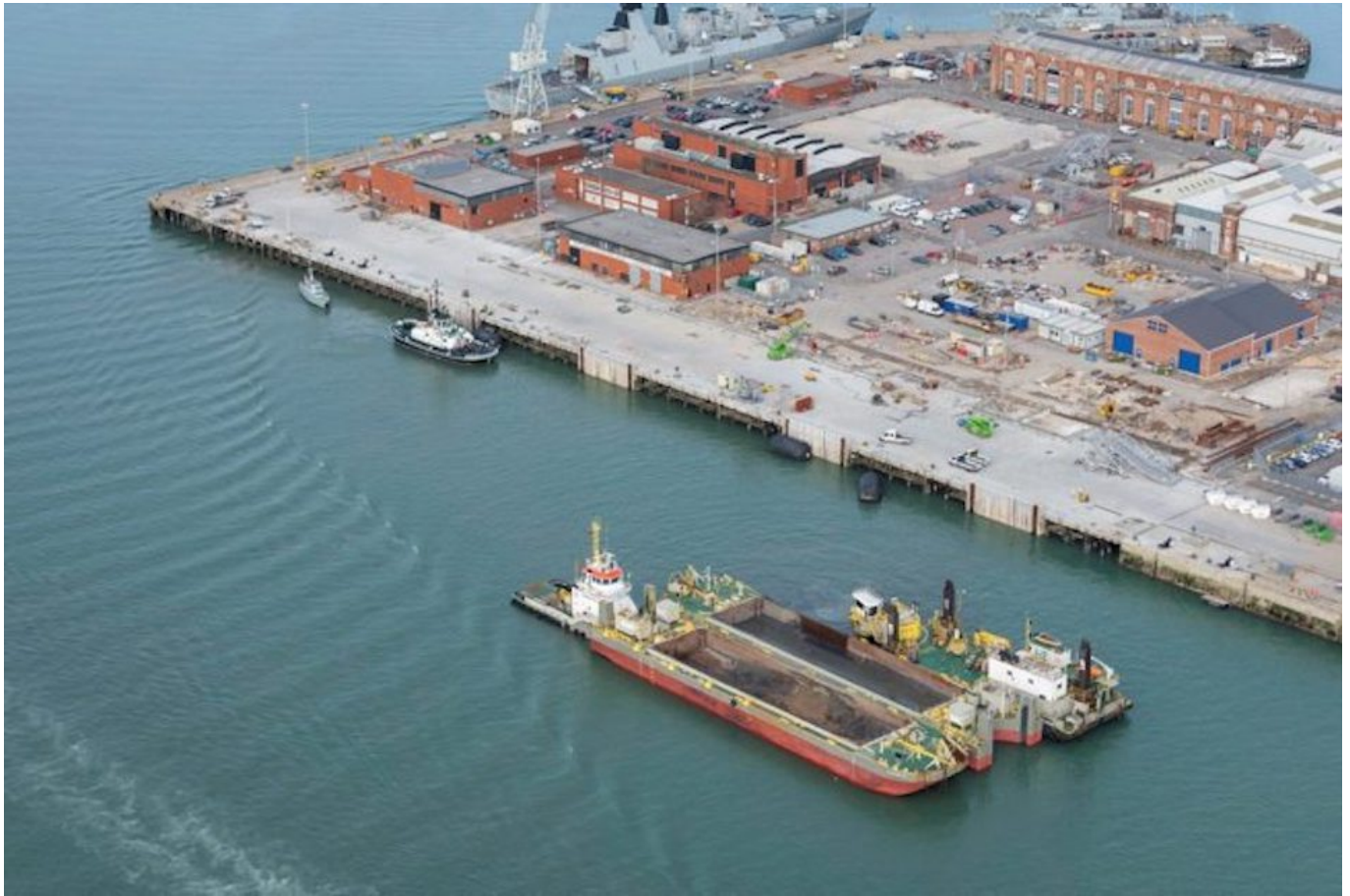
The Princess Royal Jetty from above
