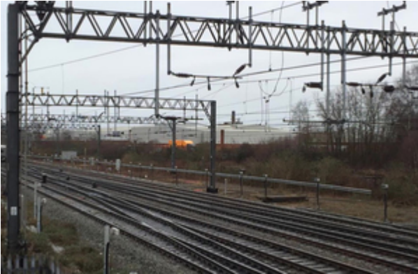
The west coast main line, Crewe
