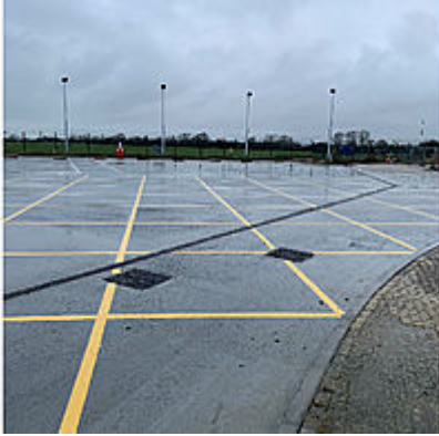
Image of the RNAS Yeovilton Bowser Park. Copyright Mott Macdonald, 2020.
