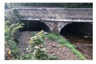
Gravel deposits have built up at the bridge and will be removed as part of the work.
