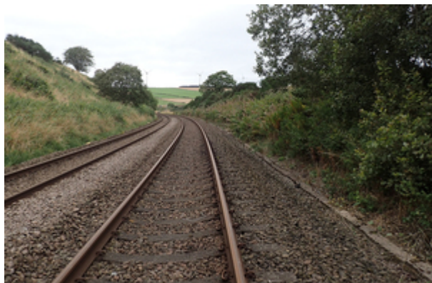
Part of the railway between Laurencekirk and Portlethen
