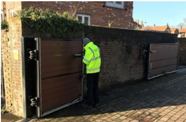
Yarm flood gates
