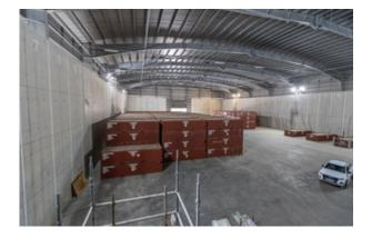
As part of the waste disposal process, the spaces between the containers in the low level waste vault are being filled with grout.
