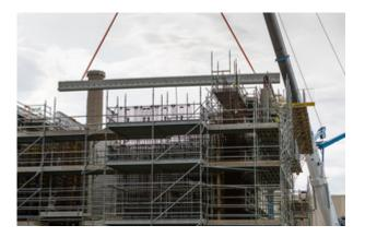
Seventy six beams, weighing a total of 1,400 tonnes, the equivalent of 116 double decker buses, are needed to complete the mammoth roof structure which will have a total weight of 3,300 tonnes. They were manufactured in Ireland and shipped to Scrabster in August.
