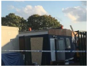
An unexpected flare from a gas gun caused one of the roofers to stumble backwards and fall from the edge of the unprotected roof to the ground below
