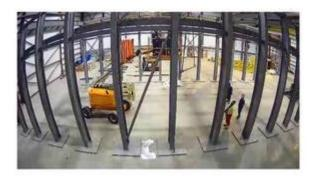
The large test frame will be used to test and trial key pieces of equipment which will then be used for decommissioning the reactor core.
