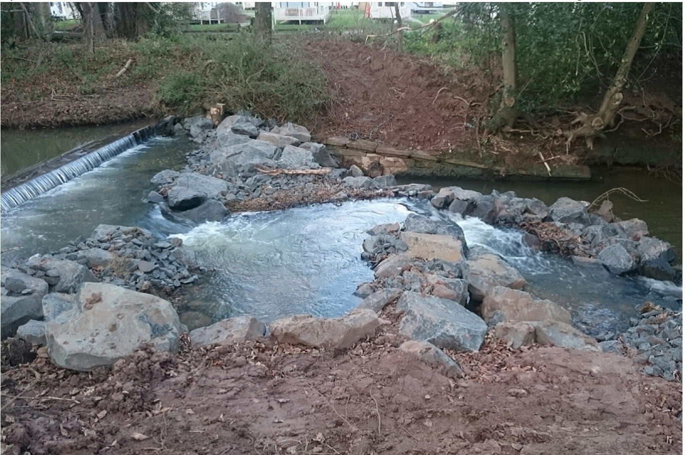
The new upstream fish pass after alterations were made to the weir to make it into a rock pass
