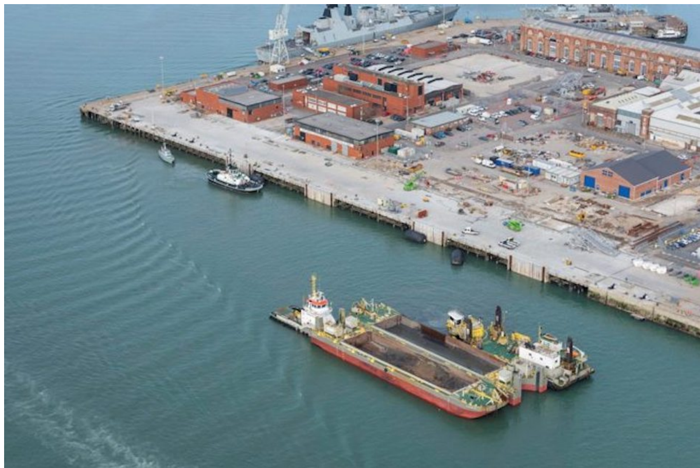
The Princess Royal Jetty from above
