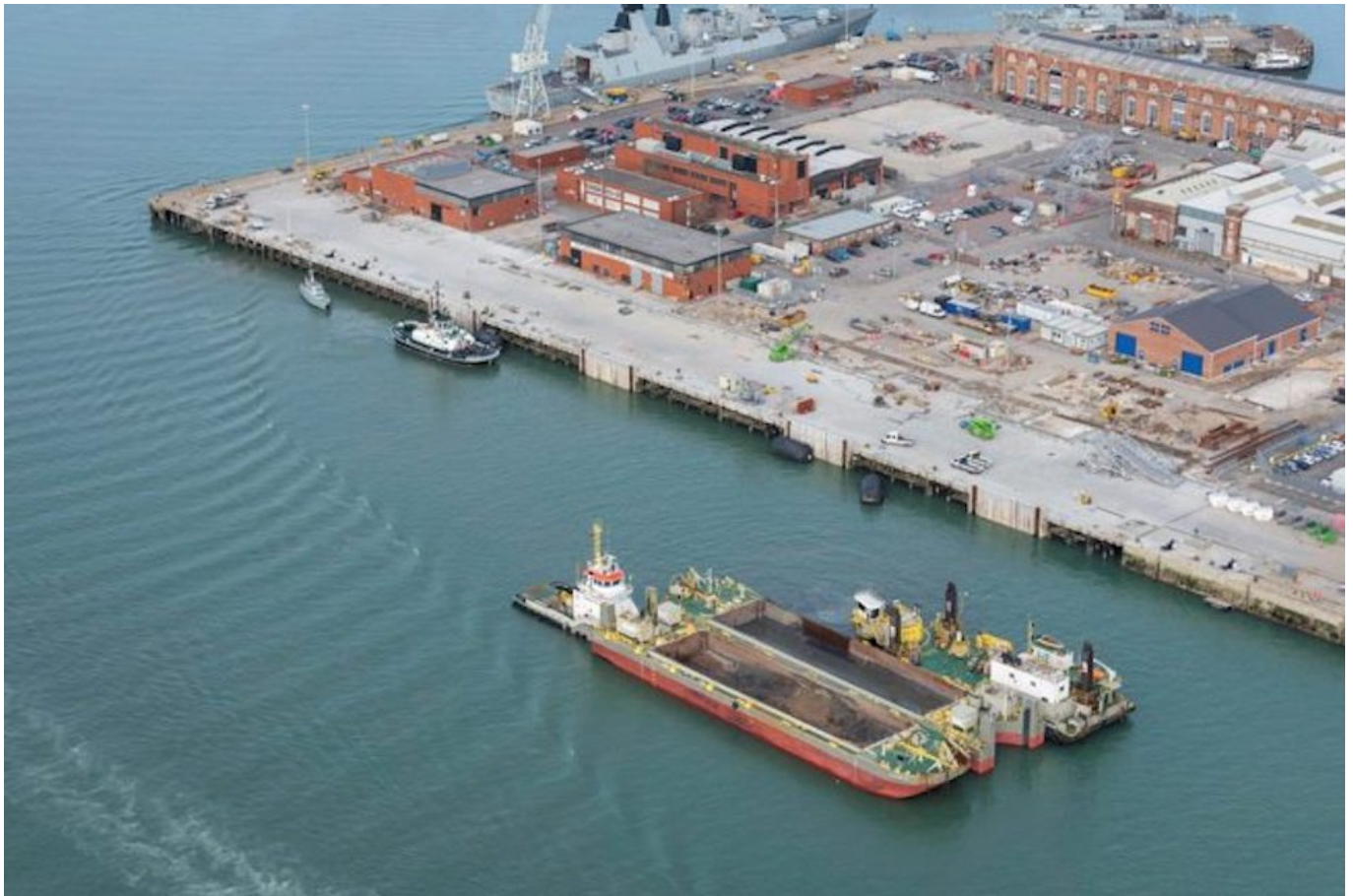
The Princess Royal Jetty from above
