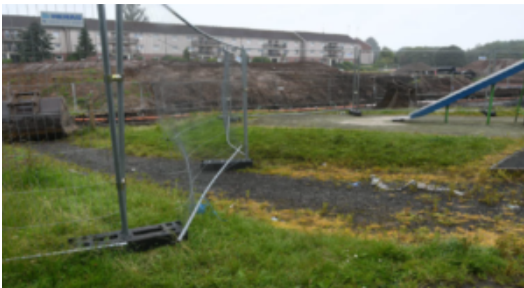
The construction site adjacent to Glenkirk Drive
