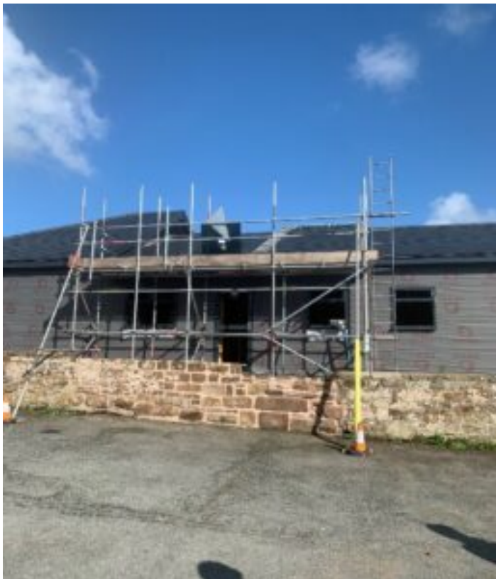
The site on Village Lane, Frodsham, Cheshire
