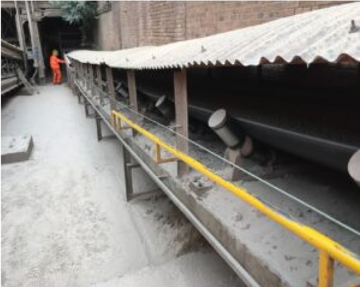
The conveyor at Mountsorrel Quarry
