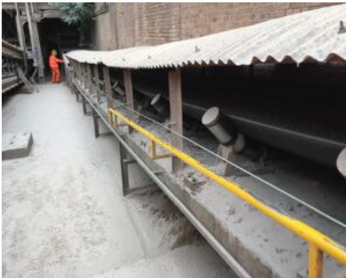
The conveyor at Mountsorrel Quarry
