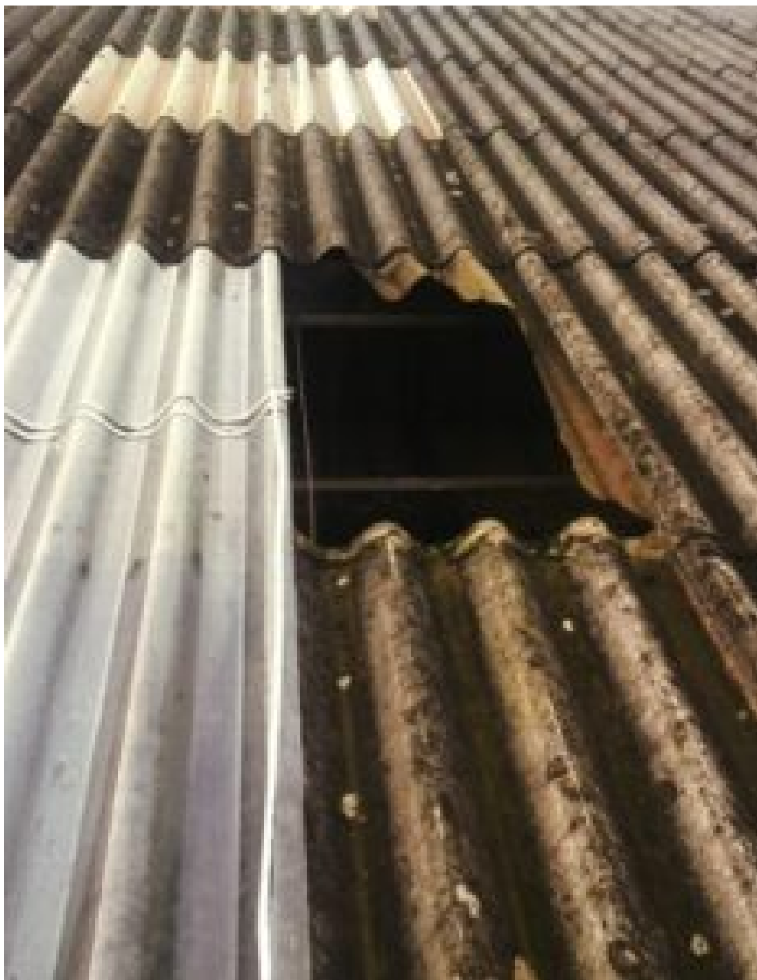
The roof Billy had been working on
