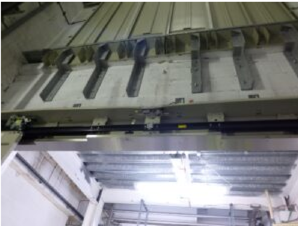
The lift shaft wall
