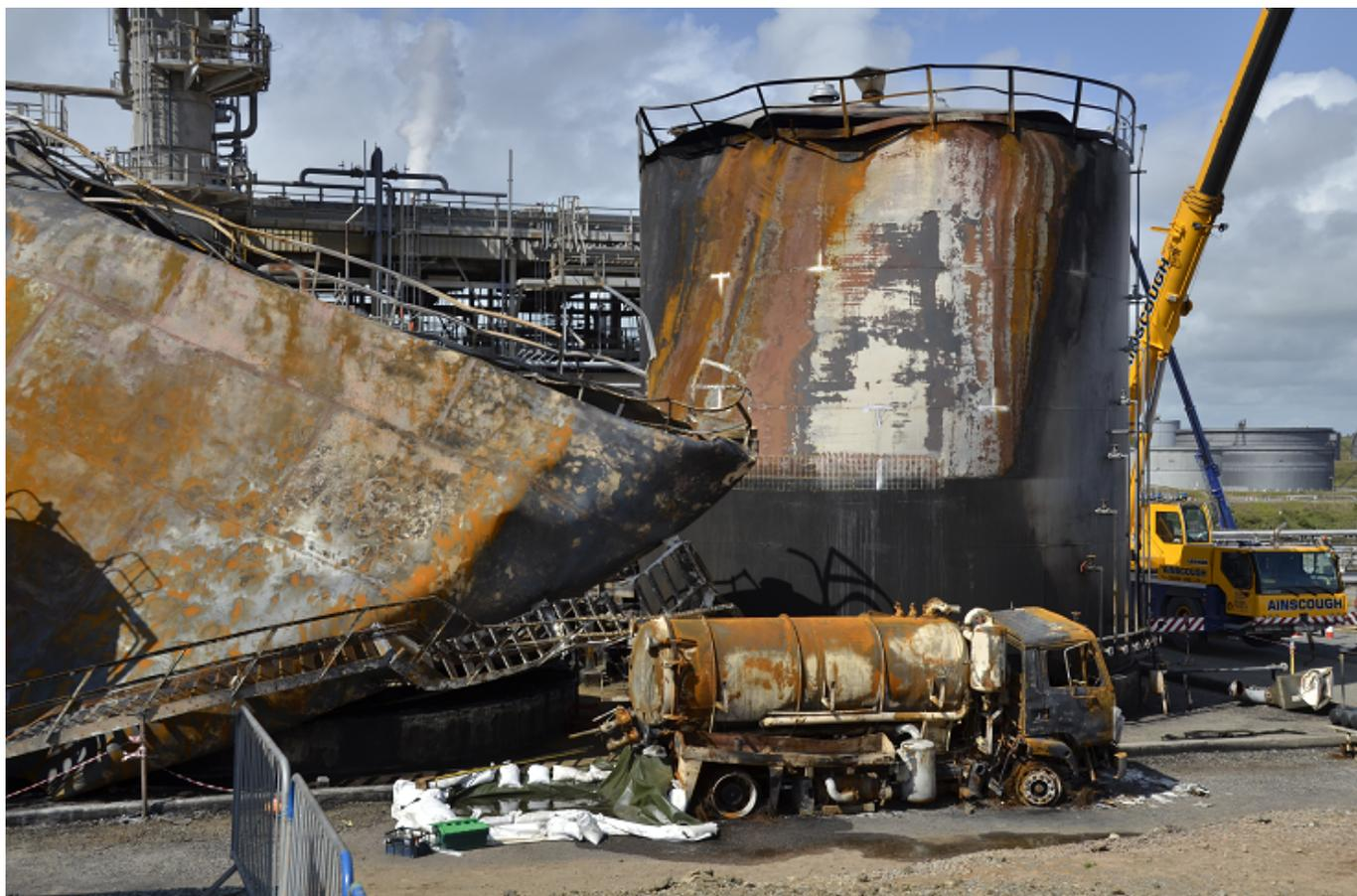
An investigation by the Health and Safety Executive found the explosion was most likely to have been initiated by the ignition of a highly flammable atmosphere within the tank, during what should have been a routine emptying operation in preparation for further cleaning and maintenance.
