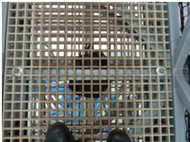
Mr Hill's trapped boot in the gangway
