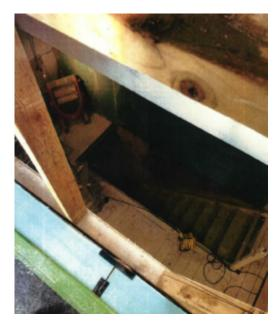
An investigation by the Health and Safety Executive (HSE) found that edge protection had been in place prior to the incident but had subsequently been removed. The company had failed to replace the edge protection before the employee was directed to carry out the work.
