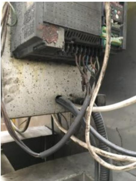
An investigation by the Health and Safety Executive (HSE) found multiple access points to dangerous parts of machinery, indicating poor maintenance of the guards. Failures in maintenance also exposed employees to live electrical conductors.
