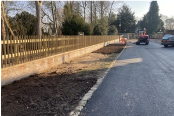
Completed flood defence wall in Bishopthorpe
