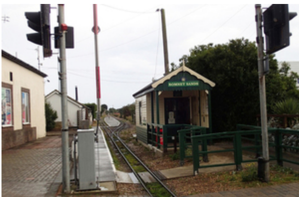
Romney Sands ticket office and station platform
