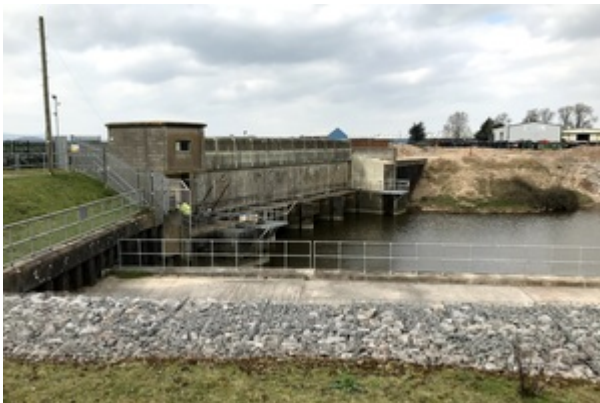
Dunball Sluice near Bridgwater
