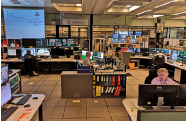
The JET control room
