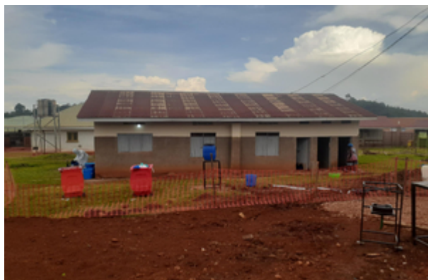
Mubende Referral Hospital Treatment Centre
