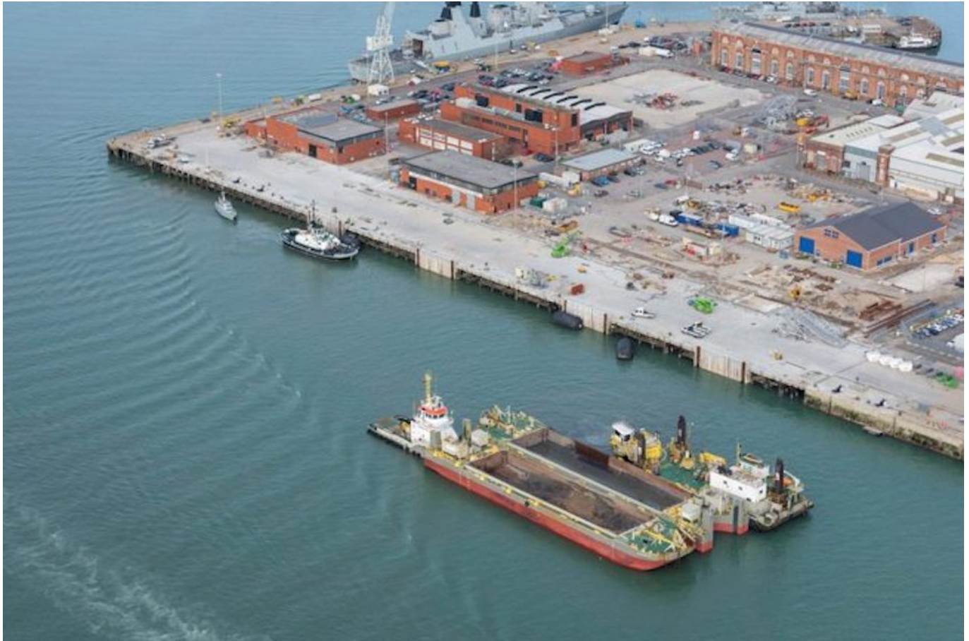
The Princess Royal Jetty from above
