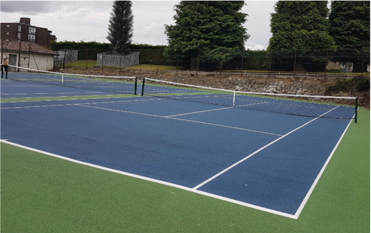
The new tennis courts are a very substantial improvement
