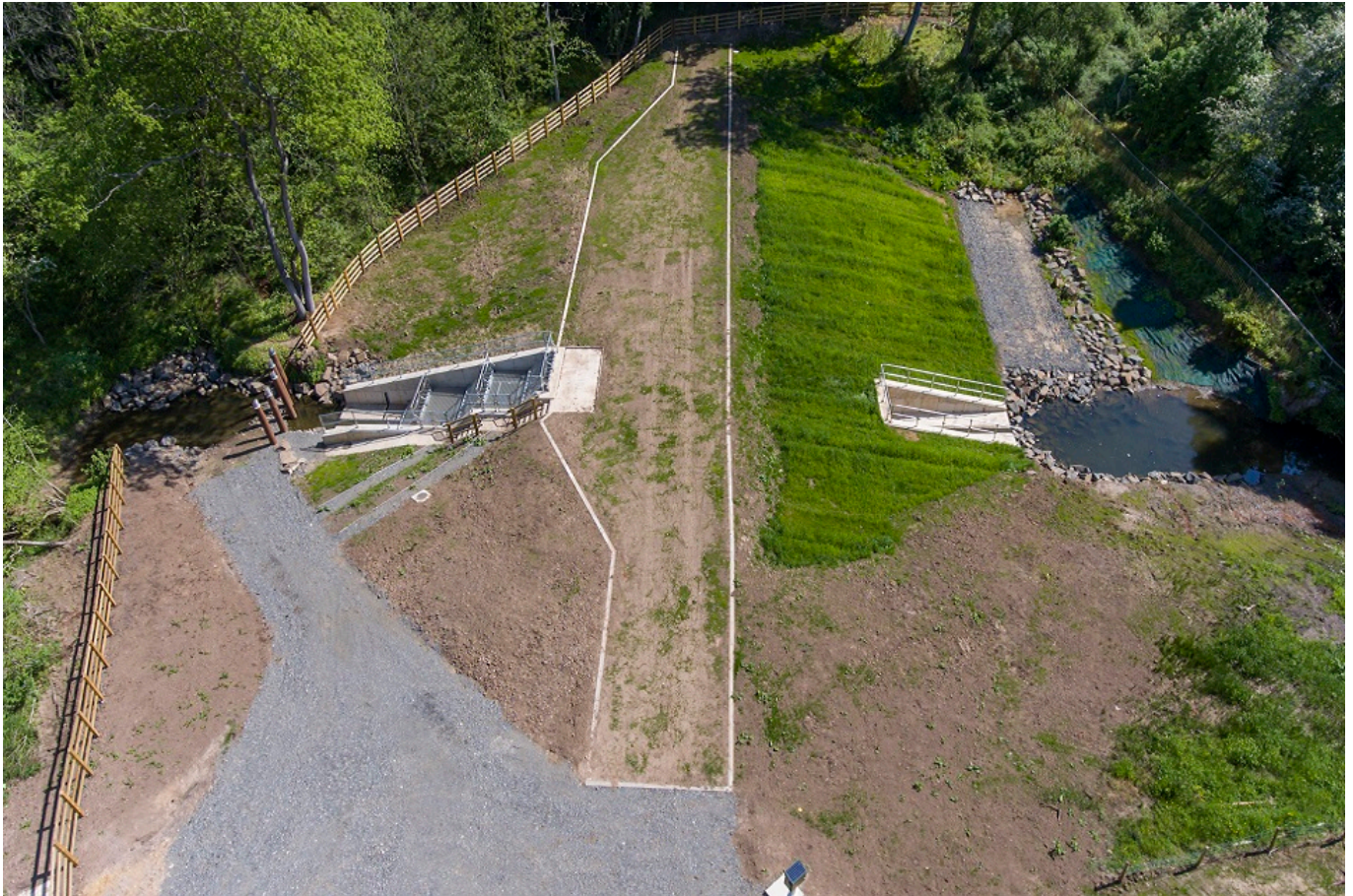
Cotting Burn dam aerial image
