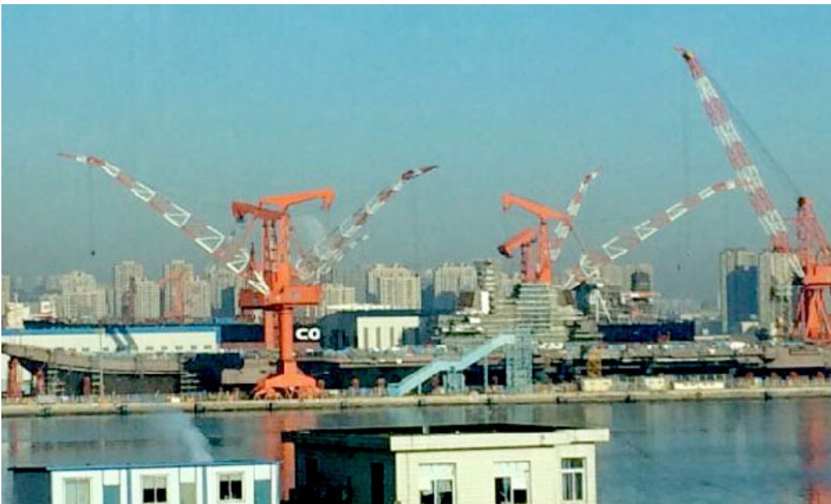
The construction site of China's first home-made aircraft carrier. [Photo/People.cn ]
