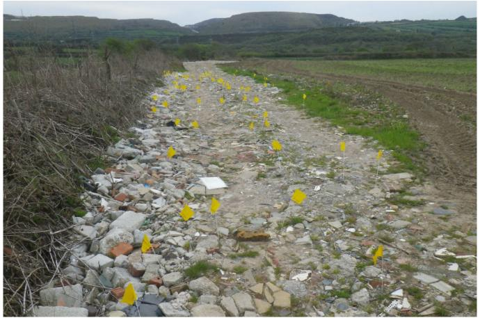
Each yellow flag in this farm track, made from waste supplied by Glebe Quarry Ltd, marks where asbestos was found
