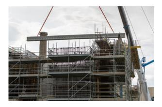
Seventy six beams, weighing a total of 1,400 tonnes, the equivalent of 116 double decker buses, are needed to complete the mammoth roof structure which will have a total weight of 3,300 tonnes. They were manufactured in Ireland and shipped to Scrabster in August.
