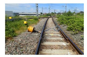
The derailment marks on the approach to Willesden High Level Junction (after track restoration)
