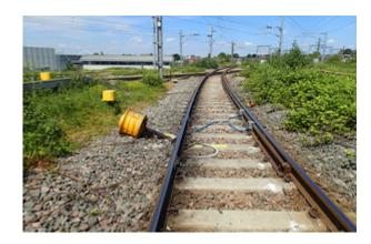
The derailment marks on the approach to Willesden High Level Junction (after track restoration)
