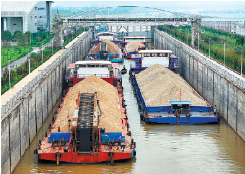
A navigation lock in operation in Xiangjiang River in Changsha, Hunan province. [Photo/Xinhua]
