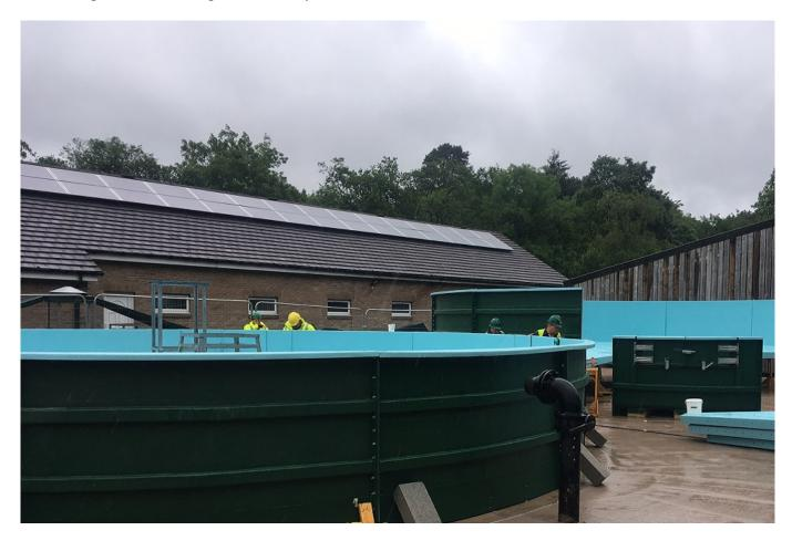
Specialist fitters were given the job of installing the £200,000 tanks on to concrete bases, specially strengthened to support the eventual 128 tonne weight of the tanks when filled.
