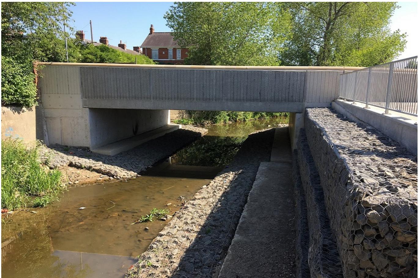
The new Londonderry Bridge
