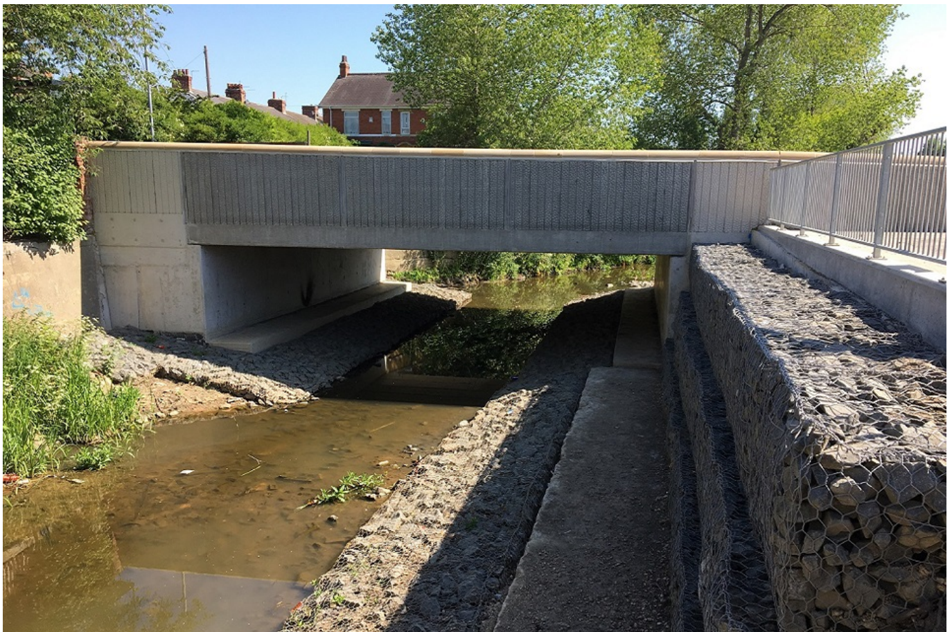
The new Londonderry Bridge
