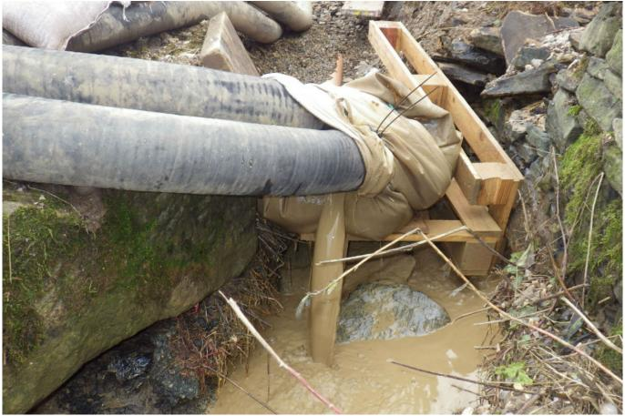
The firm's attempt to contain the muddy water was inadequate; silt was seen flowing off the site
