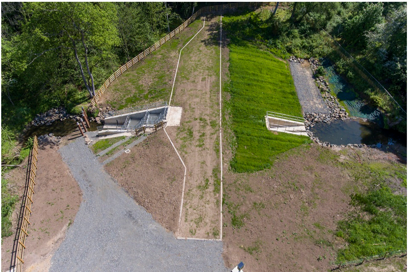
Coting Burn dam aerial image
