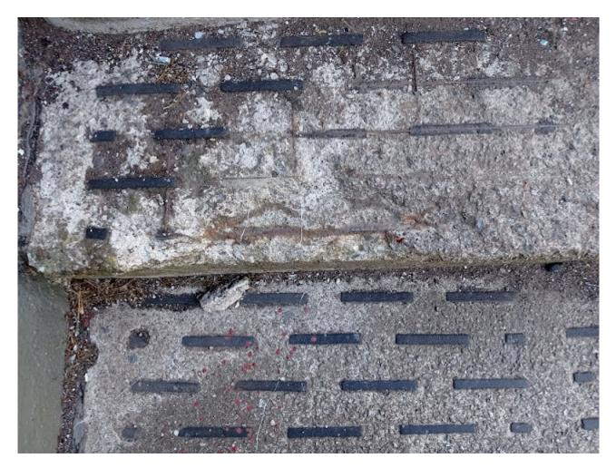
We recently received a concern that one of the steps on the footbridge over the rail line at Magdalen Green has badly worn, causing a trip hazard.
