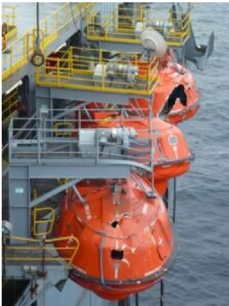
Damage to the lifeboats following the collapse
