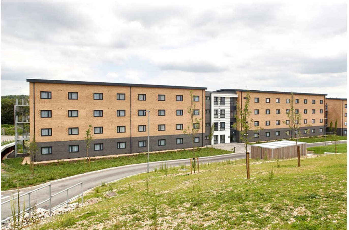
One of the SLA blocks on the site at Worthy Down. Photo courtesy of Skanska UK.
