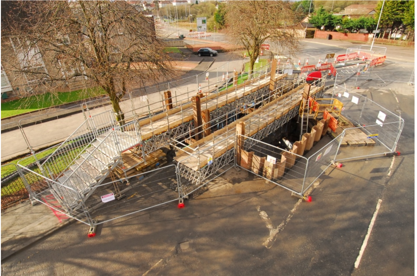
The Coal Authority's works at Kilbowie Road, Clydebank
