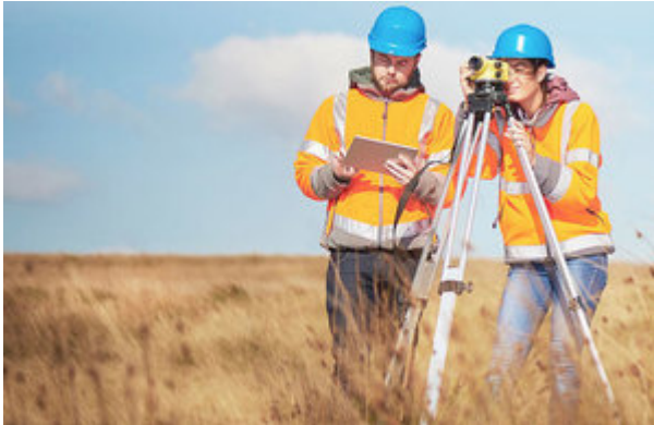
Engineers at work on a site
