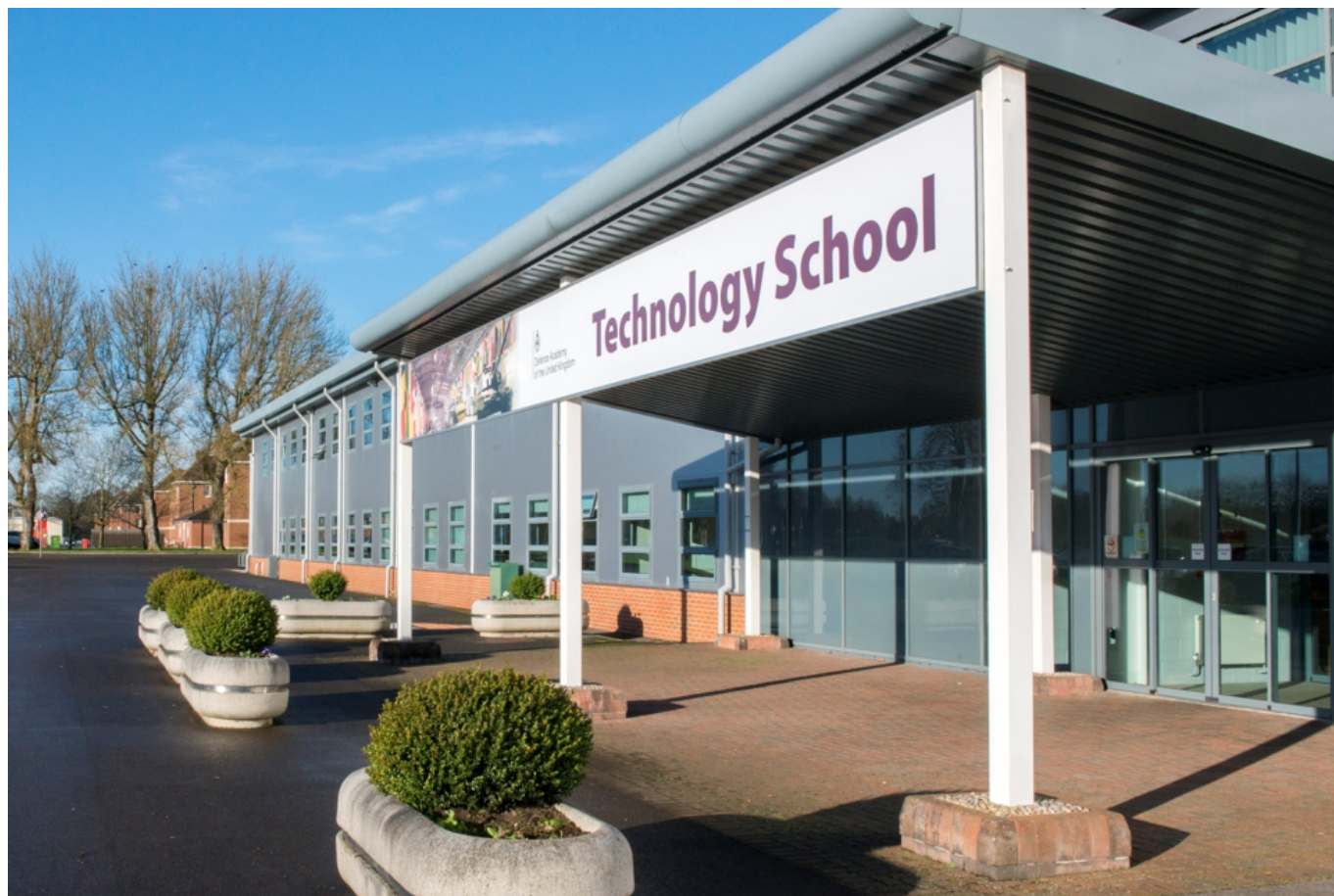
Front of the Technology School, Shrivenham
